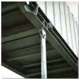
The cable exerts a force on the bracket in the direction of the cable.
