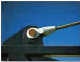
The cable exerts a force on the bracket in the direction of the cable.
