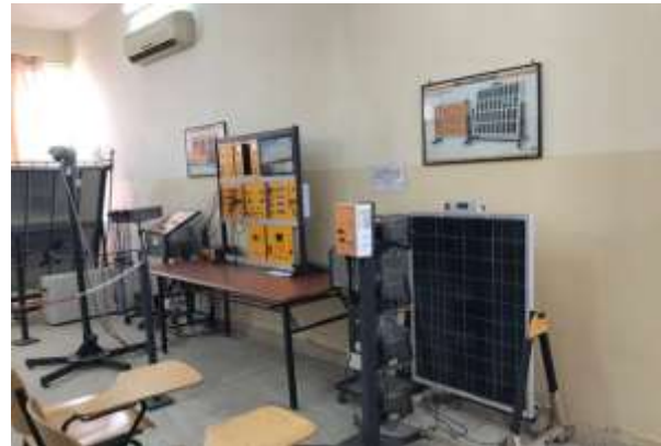
Fig. 1. Solar radiation system.
