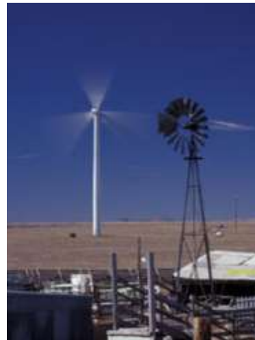
Fig. 2: a photo of a horizontal axis wind turbine
